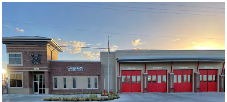
Richland Hills Fire / Rescue
