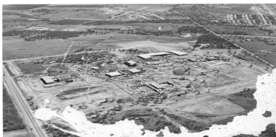
Tarrant County College Northeast Campus Construction
