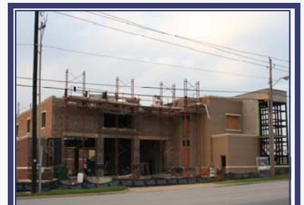
Construction of Fire Station #2
