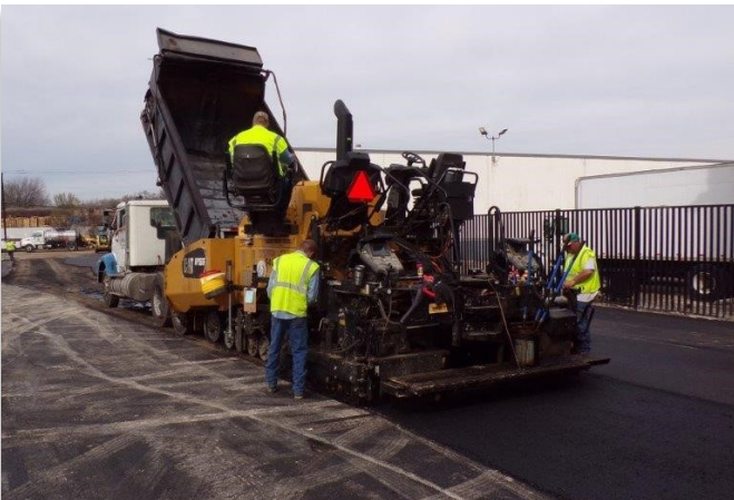
Precinct 4 workers paving a parking lot for Fort Worth ISD
