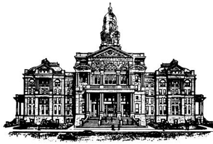
Tarrant County 1895 Courthouse
