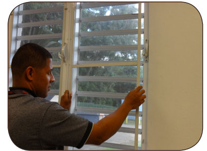
Install or repair window & door screens.
